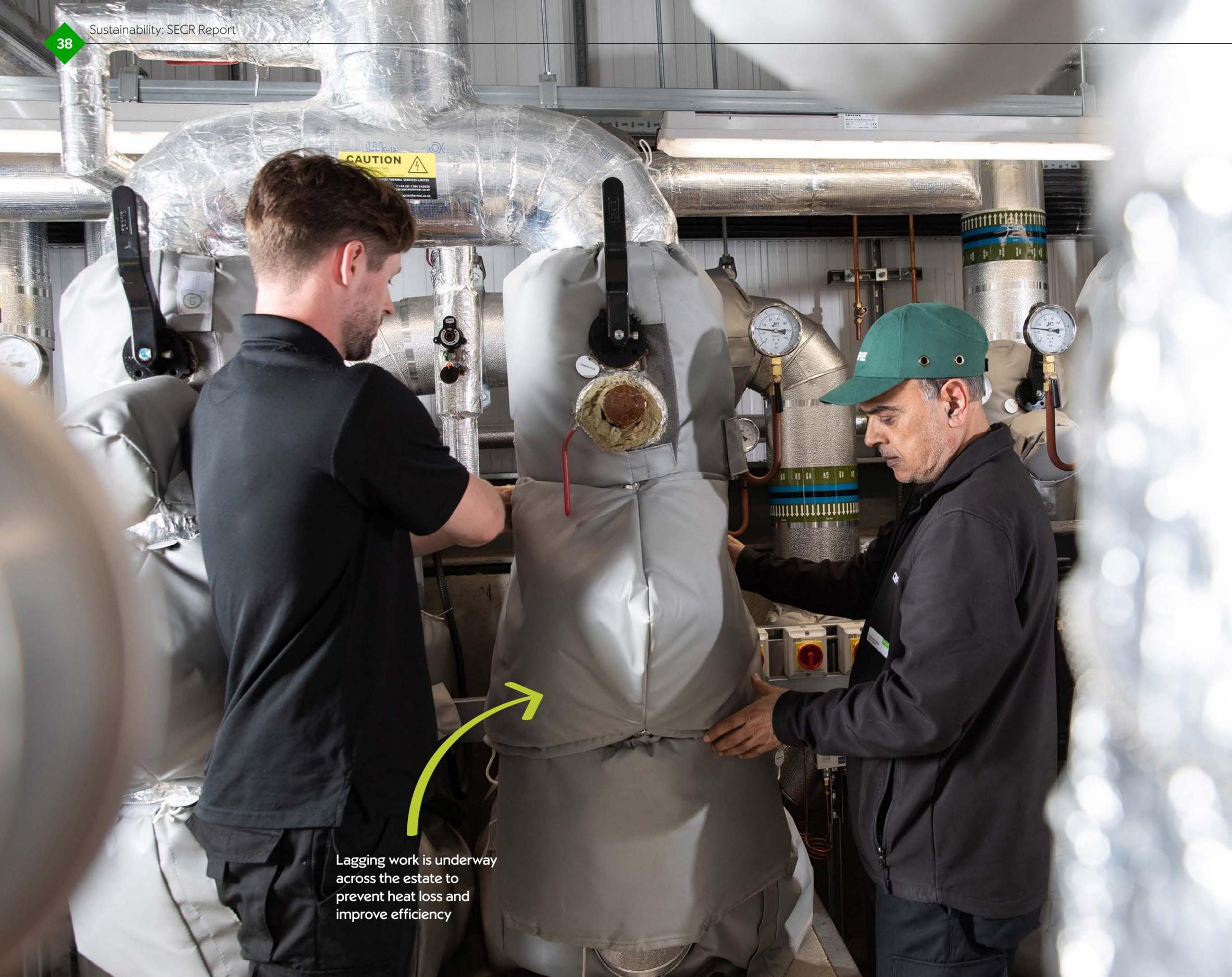
Lagging work is underway across the estate to prevent heat loss and improve efficiency
